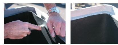
9. Replace cover into frame and install FRP reo cages before pouring concrete collar.
